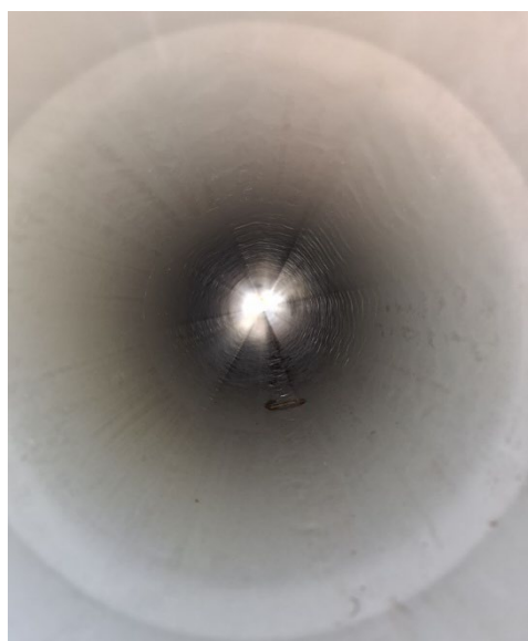
Figure 3: DN150 DWV bore rippling, photo taken at installation site with phone camera.
