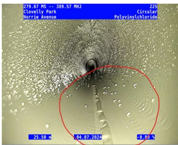
Figure 1: DN225 DWV bore rippling – CCTV view 1.
