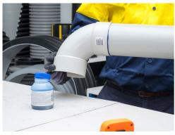
Make the joint immediately and in a single movement. Do not stop halfway, as the bond will start to set, and it will be almost impossible to insert further.
