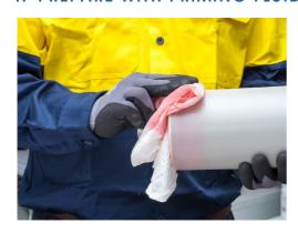
Priming fluid must be used to clean and prime all surfaces, it is vitally important to the jointing process. The priming fluid etches the PVC surface, removes the gloss, and softens for solvent cement's effective bond.
