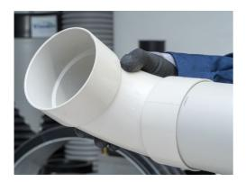
Check the spigot and socket for an interference fit by dry fitting the joint. Any adjustments can be made now, not later. An interface fit must be reached between approximately one to two thirds of the socket depth determined by the witness mark position.
