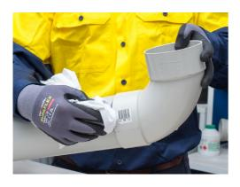
For a neat professional joint, with a clean rag, immediately wipe off excess solvent cement from the outside of the joint.
