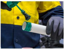
Using a suitably sized brush, apply a thin even coat of solvent cement to the internal surface of the socket first. Solvents will evaporate faster from the exposed spigot than from the socket, so the spigot should be coated last.
