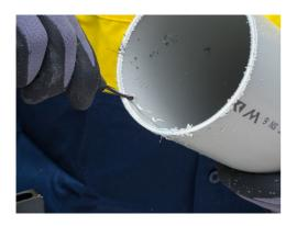
Before jointing, check that the pipe has been cut square and all the burrs are removed from the inside and outside edge. Remove the sharp edge from the outside and inside of the pipe with a deburring tool. Do not create a large chamfer that will trap a pool of solvent cement.
