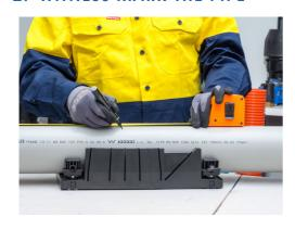
It is essential to be able to determine when the spigot is fully home in the socket. Mark the spigot with a pencil line ('witness mark') at a distance equal to the internal depth of the socket.
