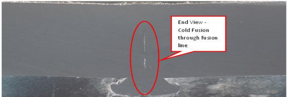
CROSS-SECTIONAL VIEW FROM DESTRUCTIVE VERIFICATION OF COLD FUSION IN BF JOINT
