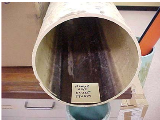
Figure 1. Sulphide staining at invert.
