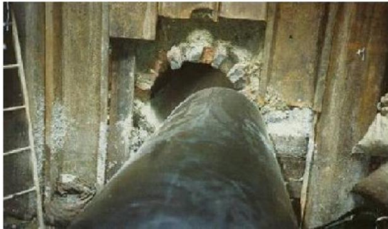
PE LINER ABOUT TO ENTER AN OLD BRICK SEWER – PHOTO COURTESY OF VINIDEX
