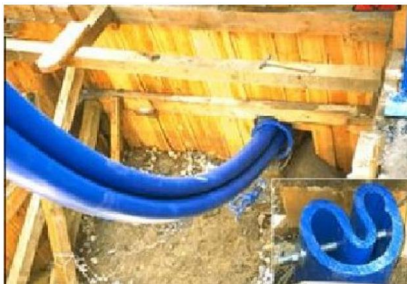
“COMPACT PIPE”, INSERT SHOWING CROSS-SECTIONAL SHAPE
