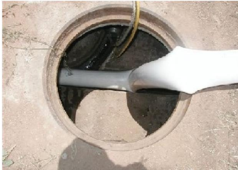
“EX” PIPE PVC LINER SYSTEM ENTERING A SEWER ACCESS CHAMBER – COURTESY OF VINIDEX
