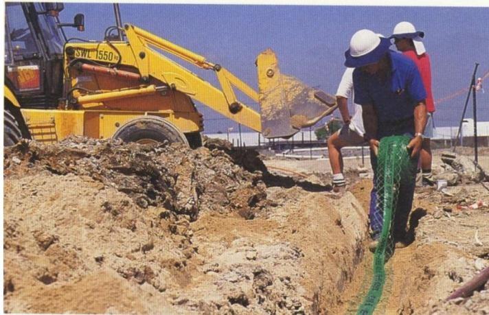
*Marker tape being installed in the trench above the pipe
